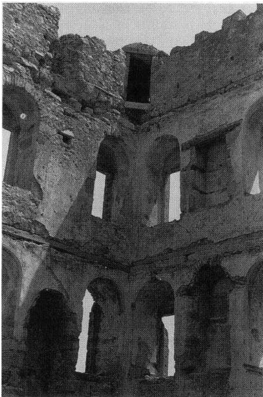
Figure 4.6. Çanakkale Cezayirli Hasan Paga Köskü, interior. All the stretchers were cut in Spring 1783. (P. I. Kuniholm, ADP)
